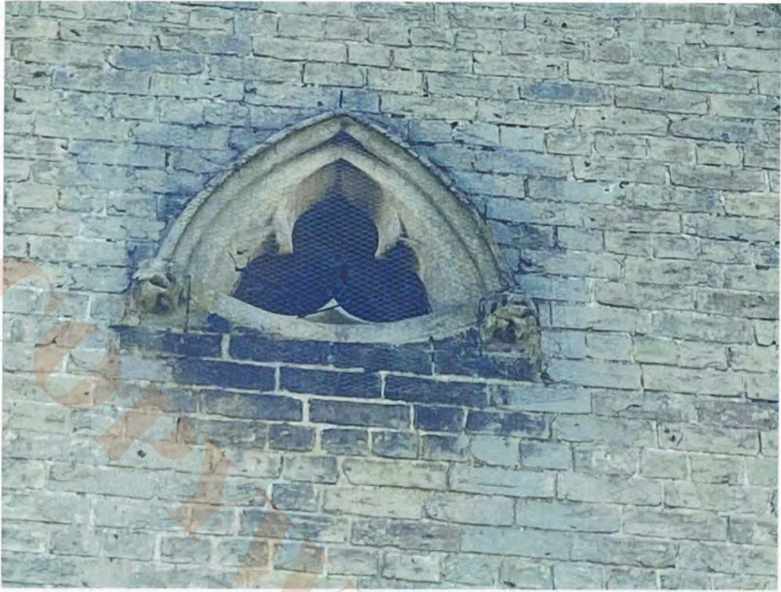
9.26 North chapel east high level opening
