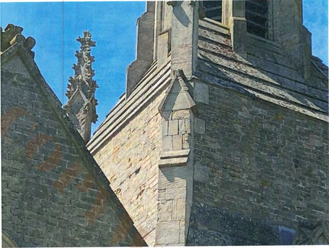
8.6 Tower south east buttress
