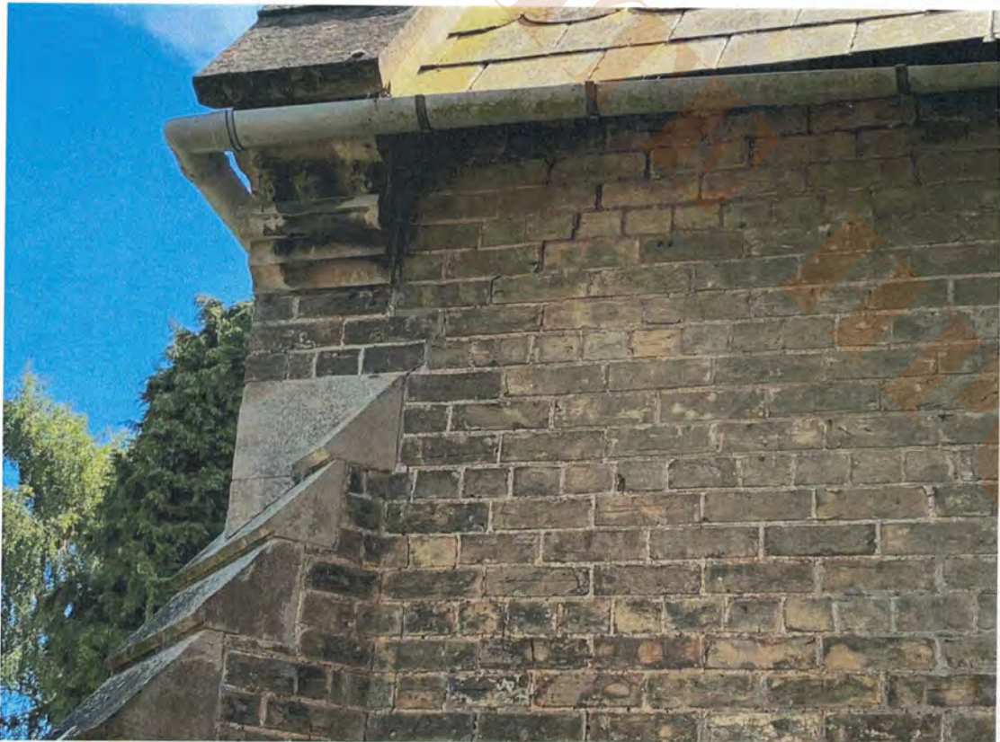
8.37 South chapel north elevation east of tower
