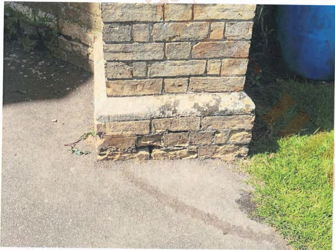
8.20 North chapel south east buttress
