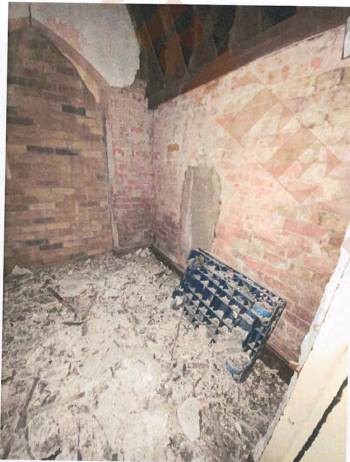
11.18 South porch floor
