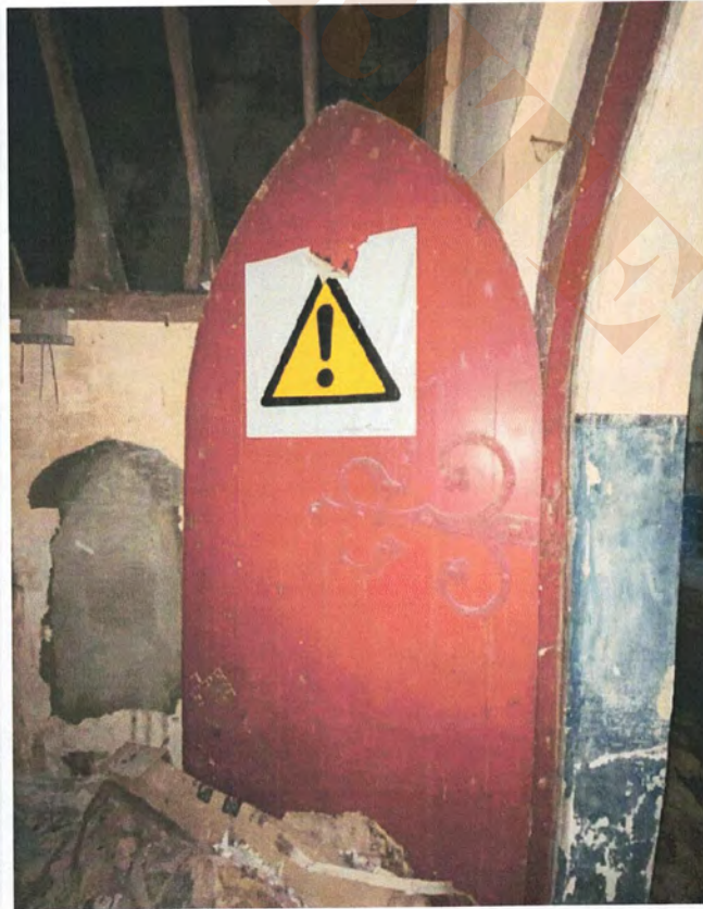
11.32 North porch interior door
