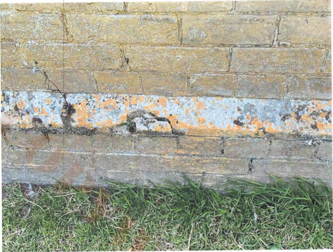
8.21 North chapel east plinth offset
