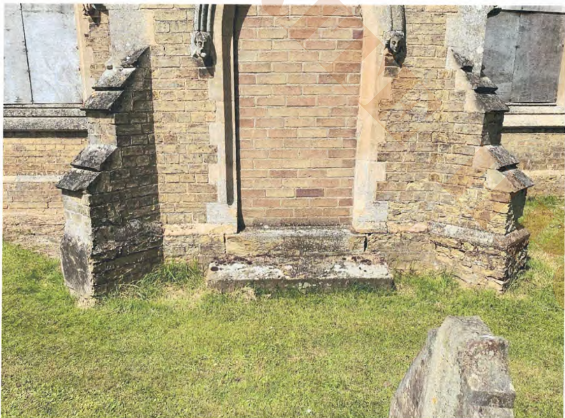
8.57, 8.58 South porch south elevation
