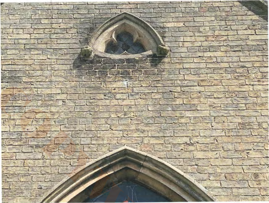
8.28 North chapel west elevation
