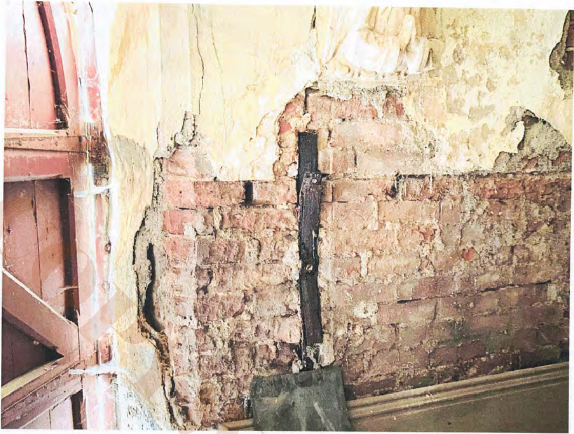
11.37 North chapel south wall ironwork
