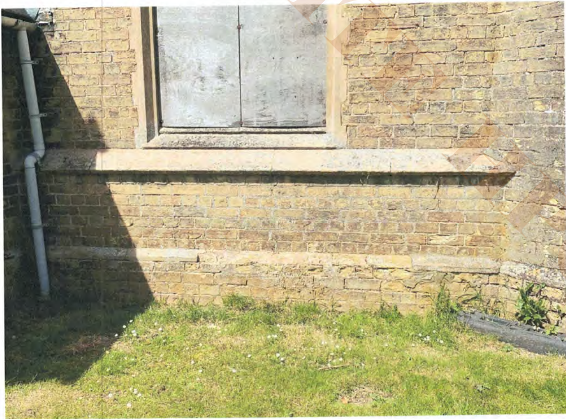
8.46, 8.47 South chapel south elevation east of porch
