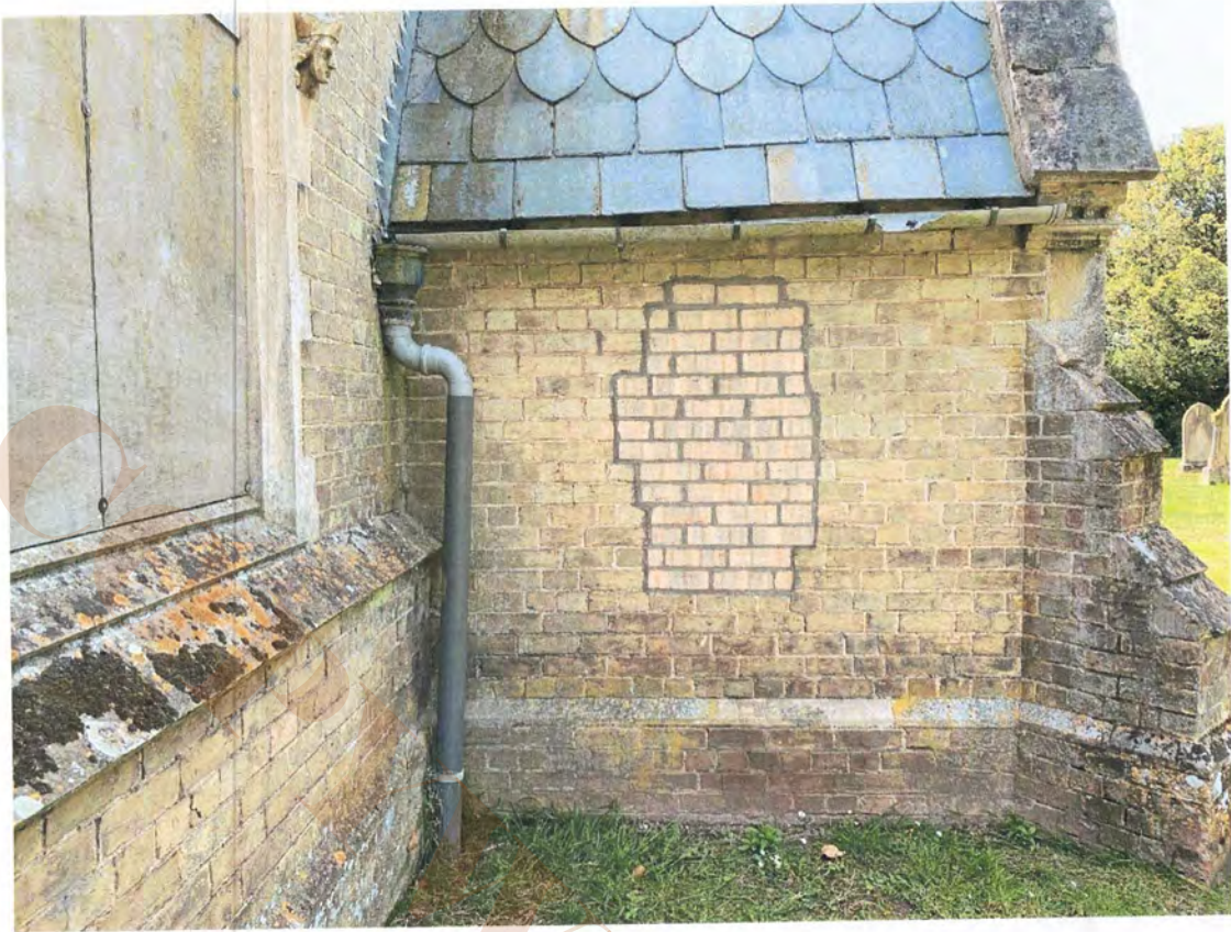
10.4 North porch west eaves
