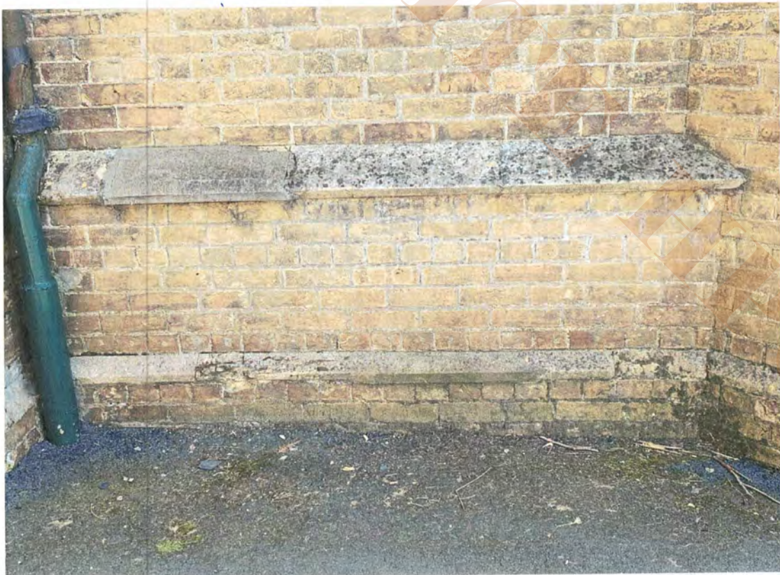
8.39 South chapel north elevation west of tower: plinth
