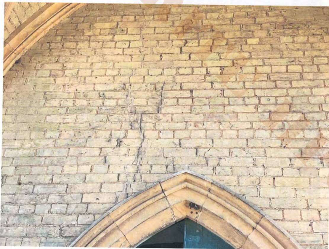
11.9 Carriageway north wall
