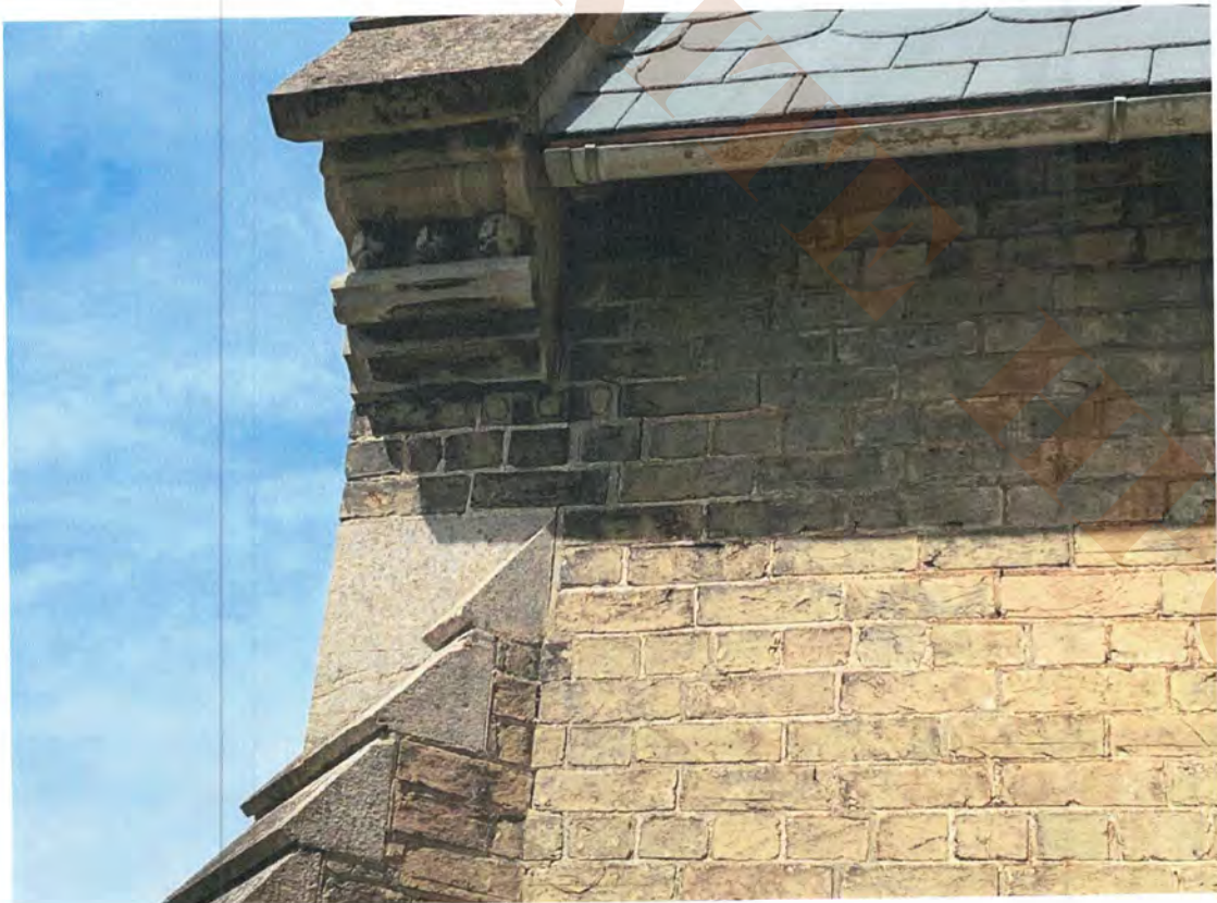
8.25 North chapel south elevation west of tower
