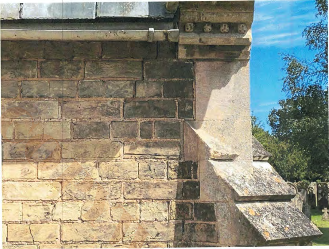
8.59 South porch west elevation
