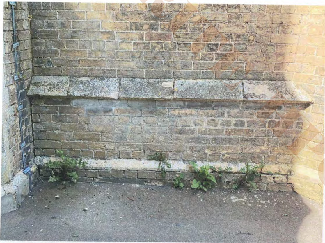
8.23 North chapel south elevation east of tower: plinth
