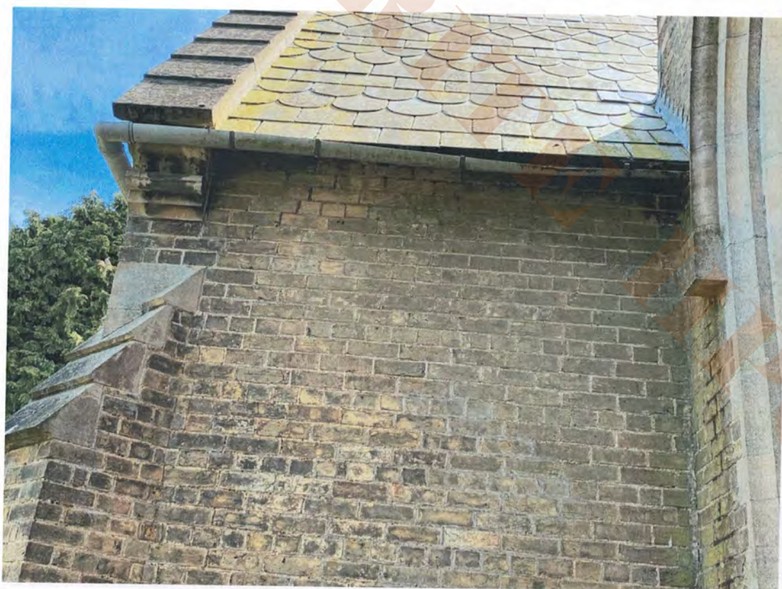
10.9 South chapel north rainwater goods east of tower
