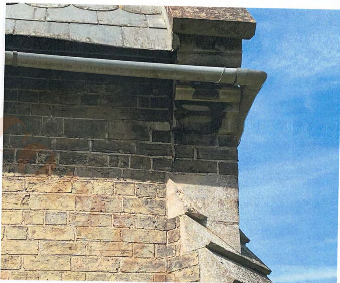
8.47 South chapel south elevation east of porch
