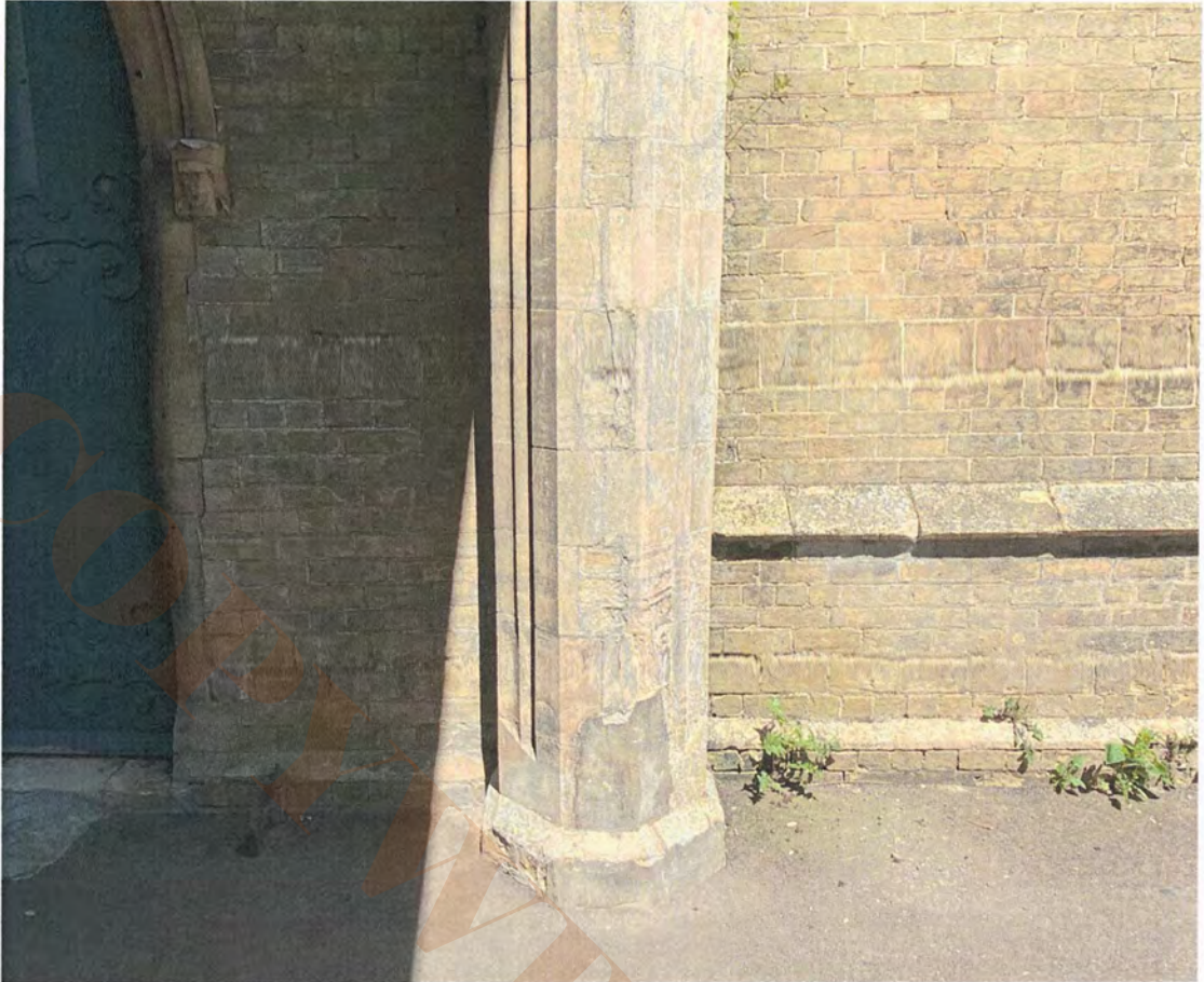
9.7, 9.8 Tower east elevation north pier
