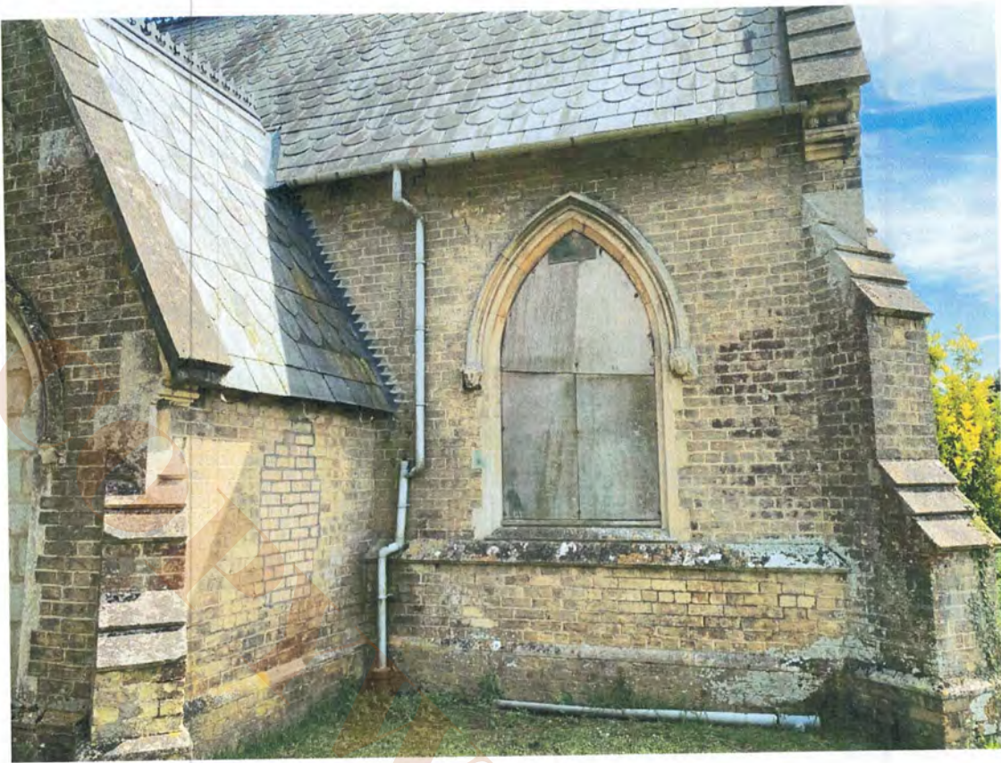
10.2 North chapel rainwater goods: west of the porch
