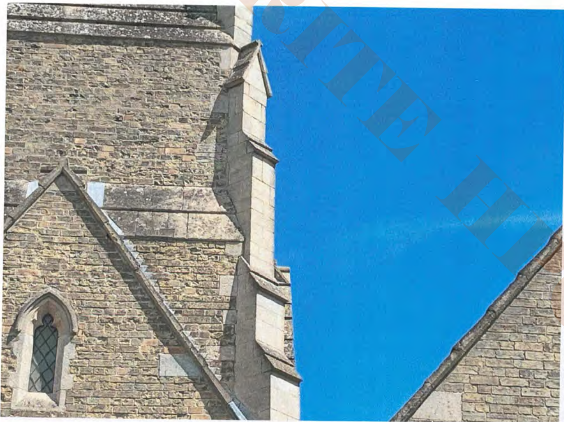
8.13 Tower west elevation triangular panels
