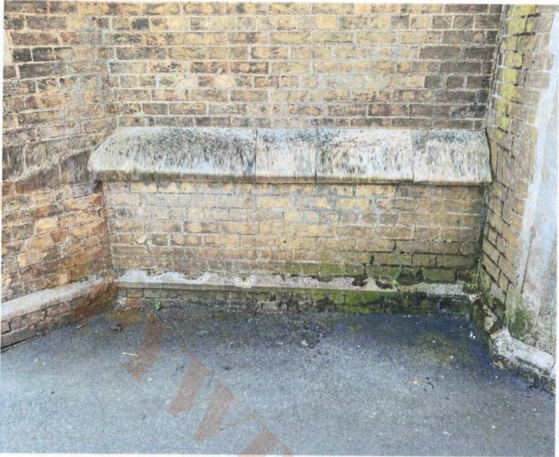
8.36 South chapel north elevation east of tower
