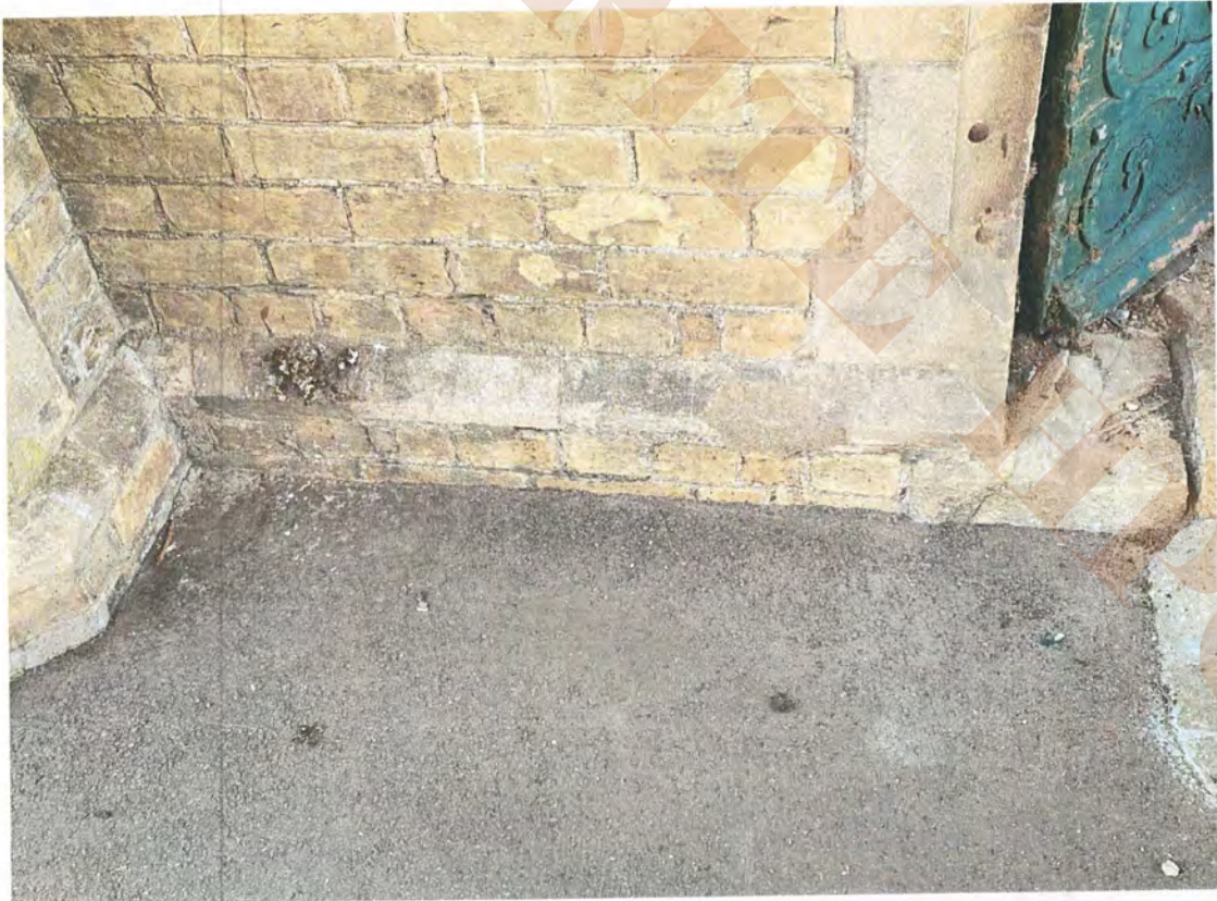
11.10 Carriageway north plinth
