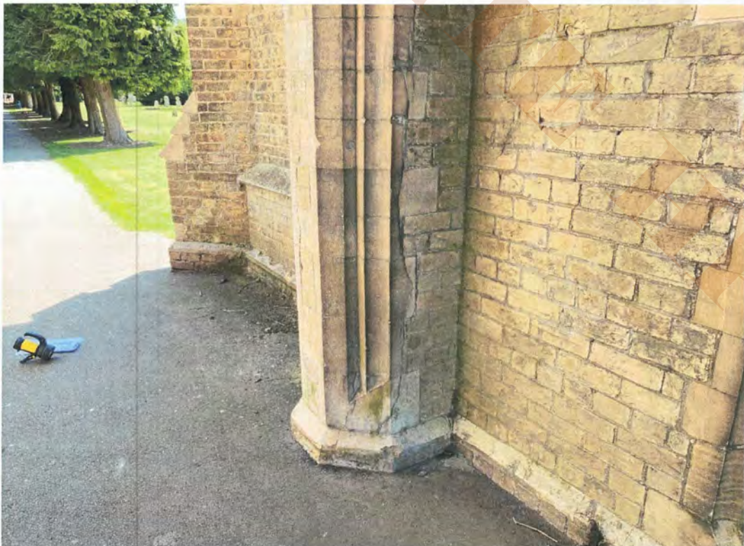
9.6 Tower east elevation south pier
