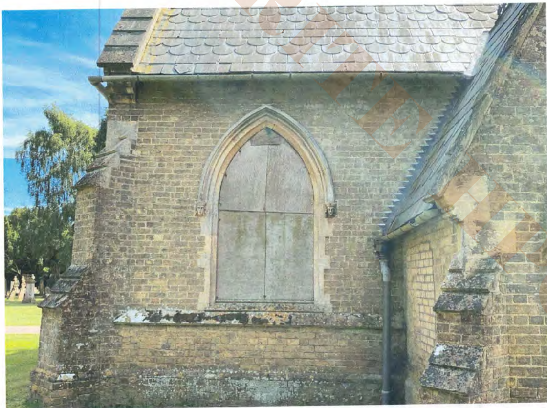
10.3 North chapel rainwater goods: east of porch
