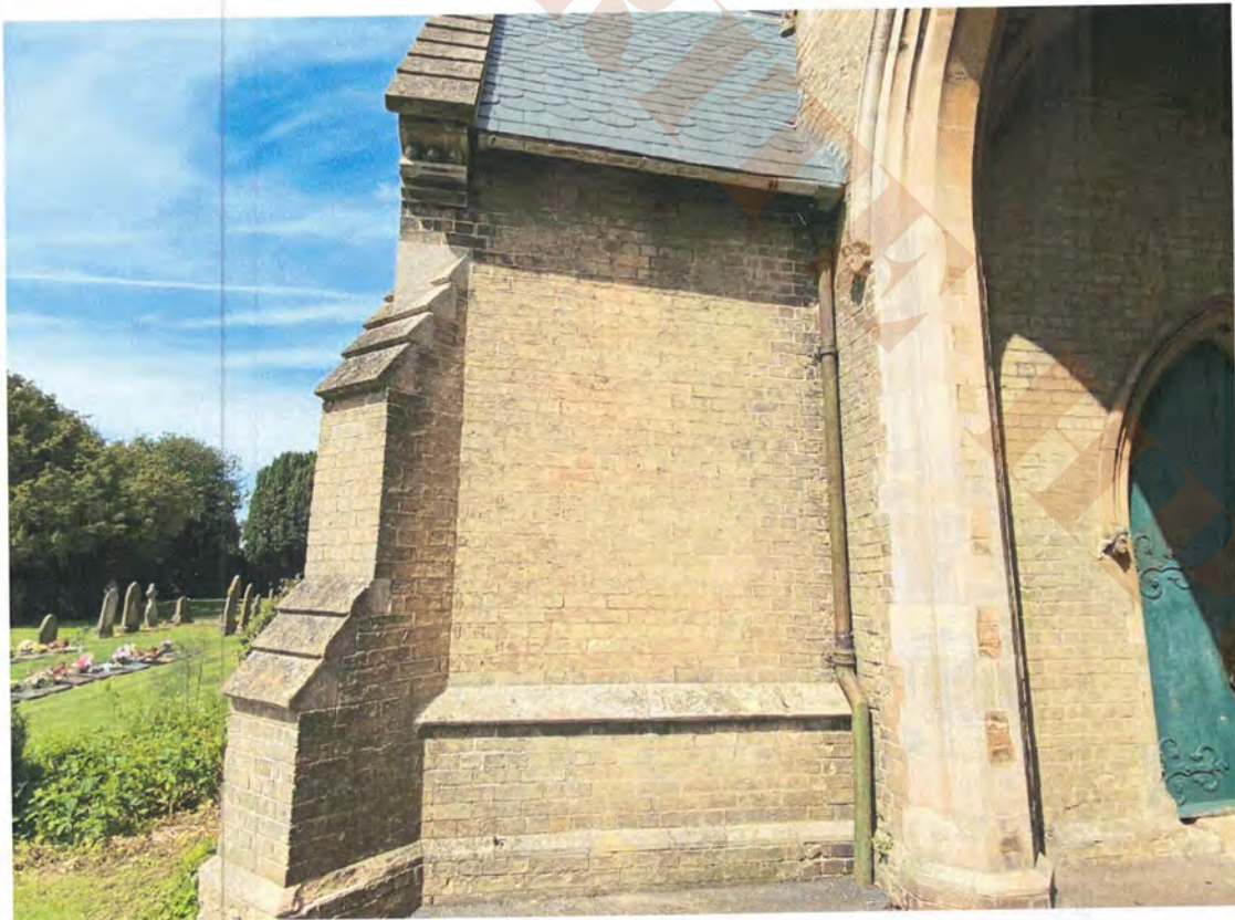
10.5 North chapel south eaves rainwater goods: west of tower
