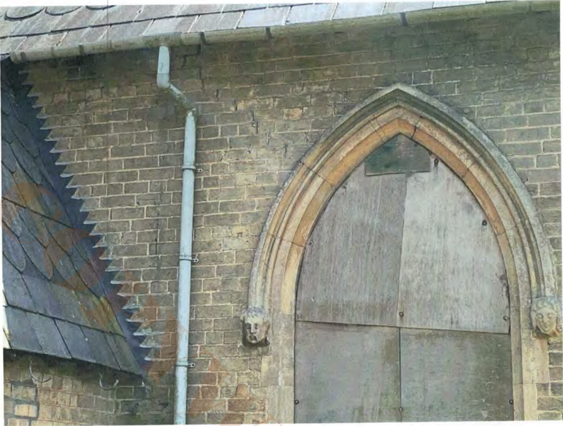
8.19 North chapel north elevation west of porch
