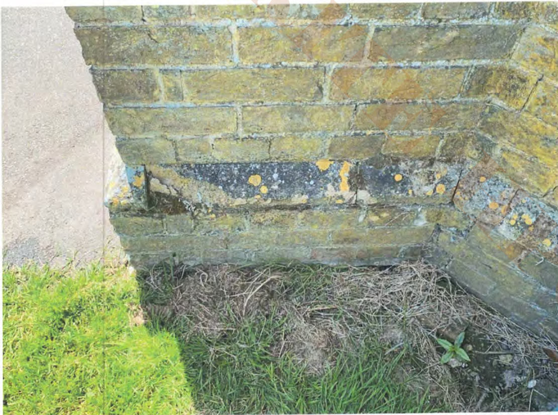
8.21 North chapel south west buttress plinth offset
