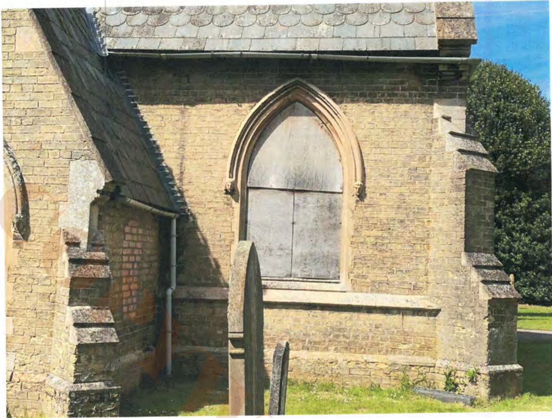
10.10 south chapel south rainwater goods east of porch
