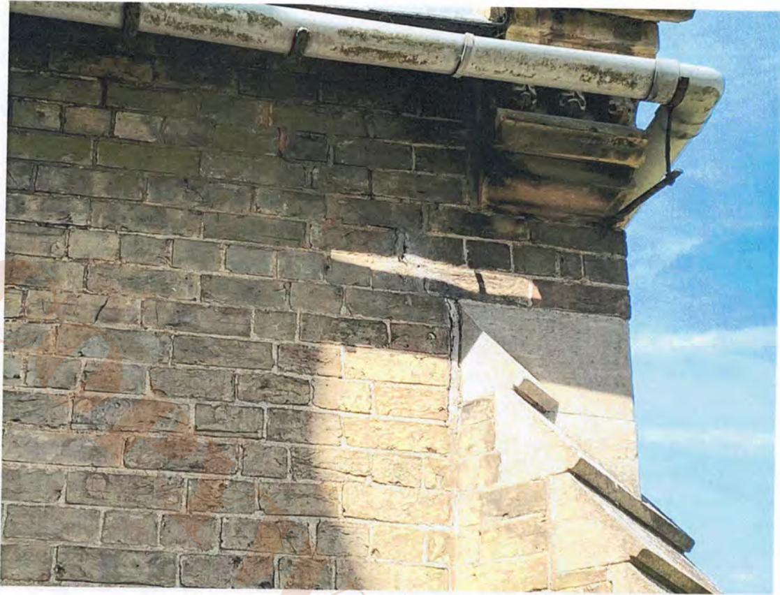
8.22 North chapel south elevation east of tower
