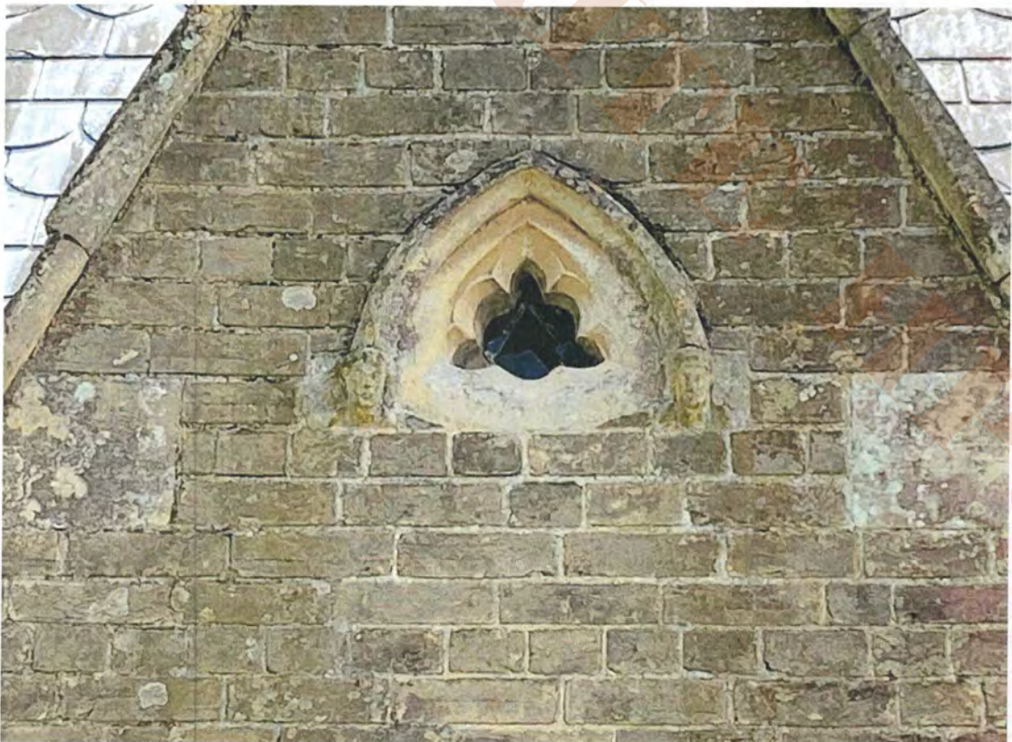
9.14 North porch north gable high level opening
