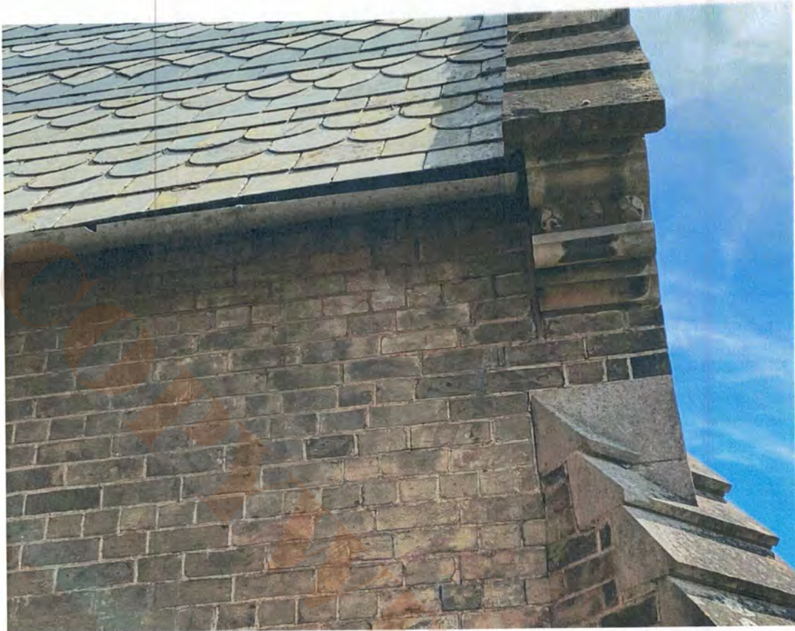
8.38 South chapel north elevation west of tower
