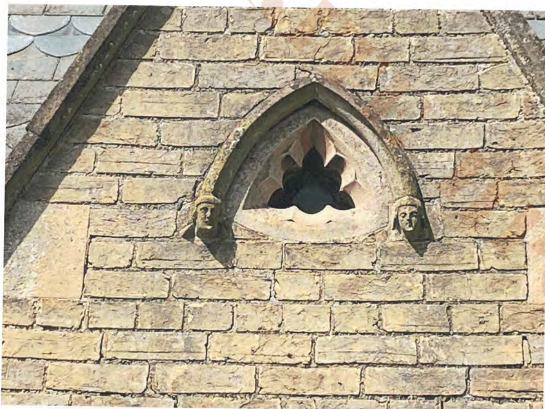
9.41 South porch south gable opening
