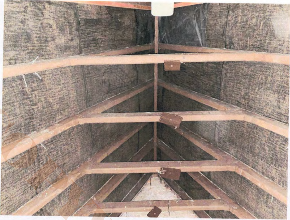
11.17 South porch ceiling
