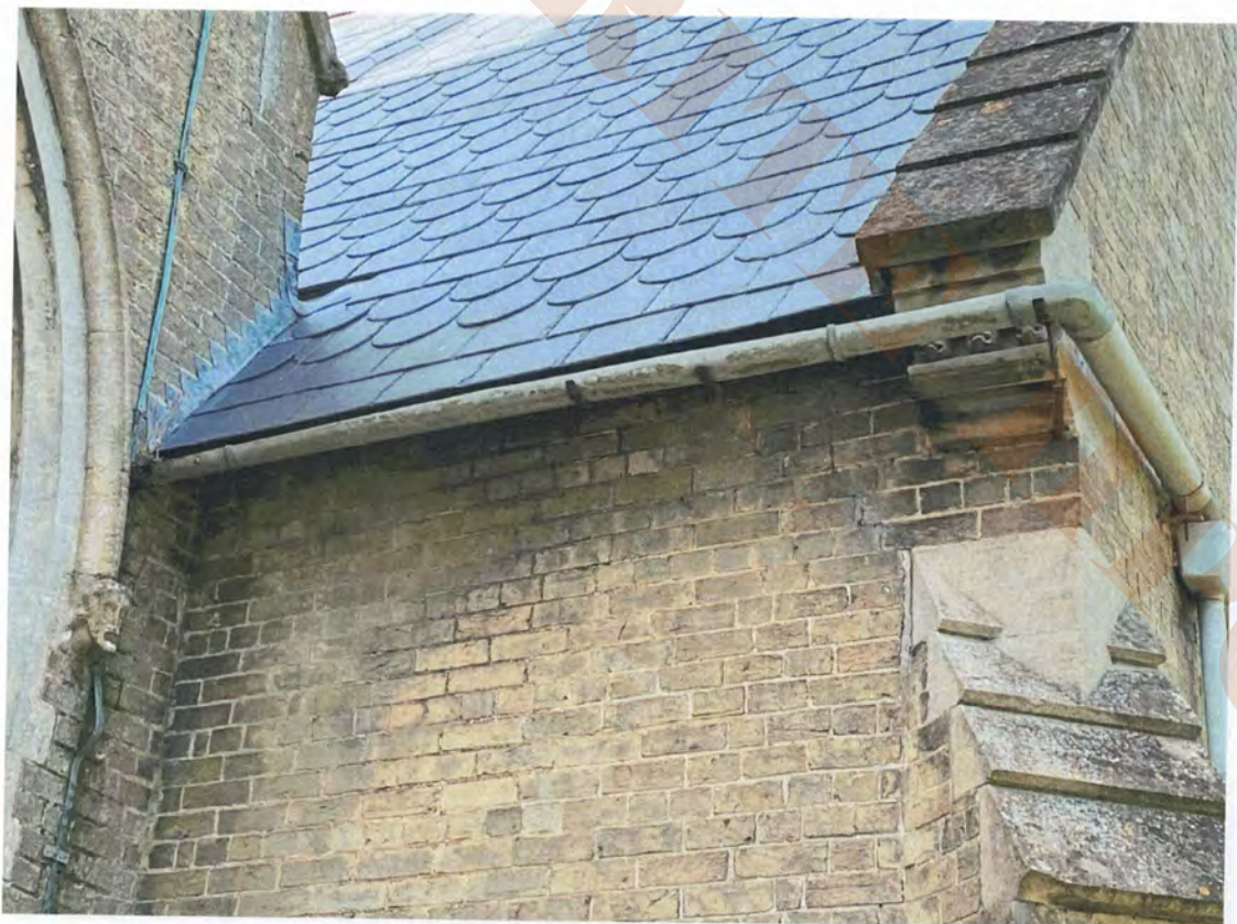
10.4 North chapel rainwater goods: south eaves east of tower
