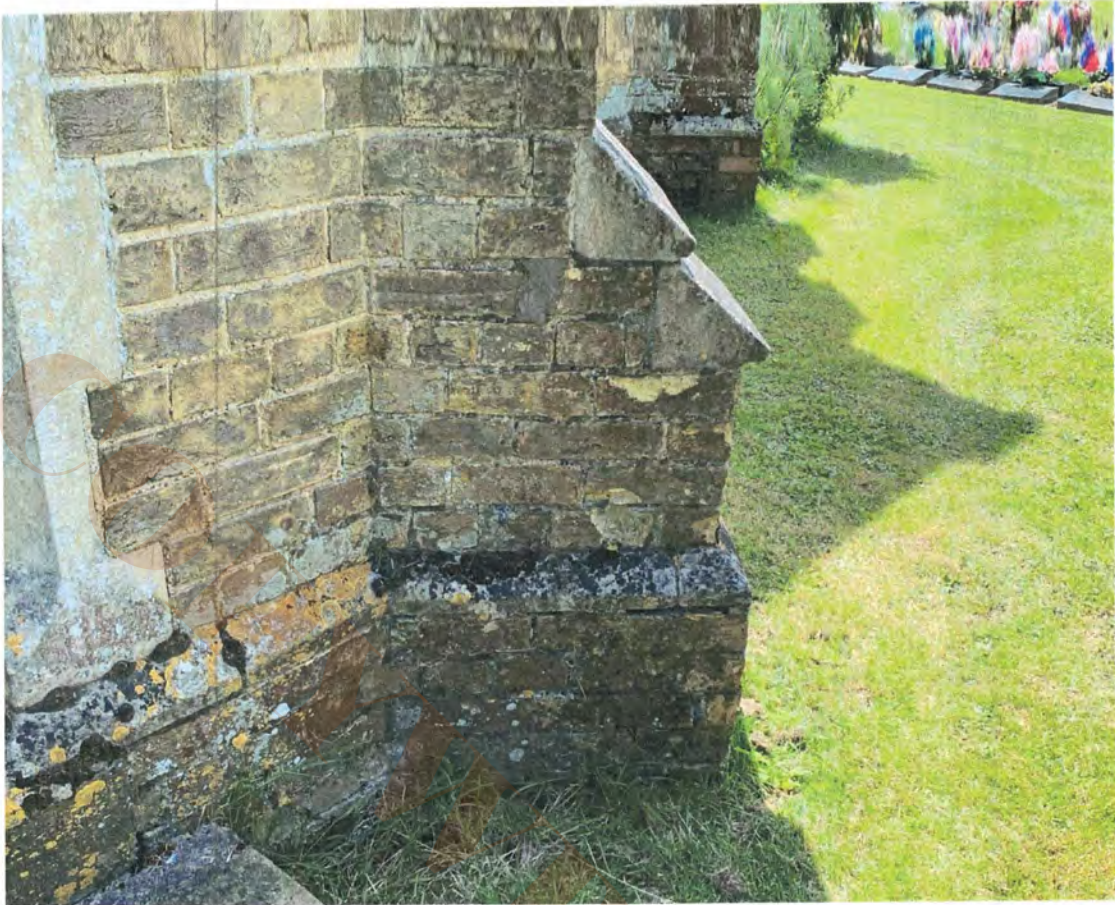
8.33 North porch north west buttress
