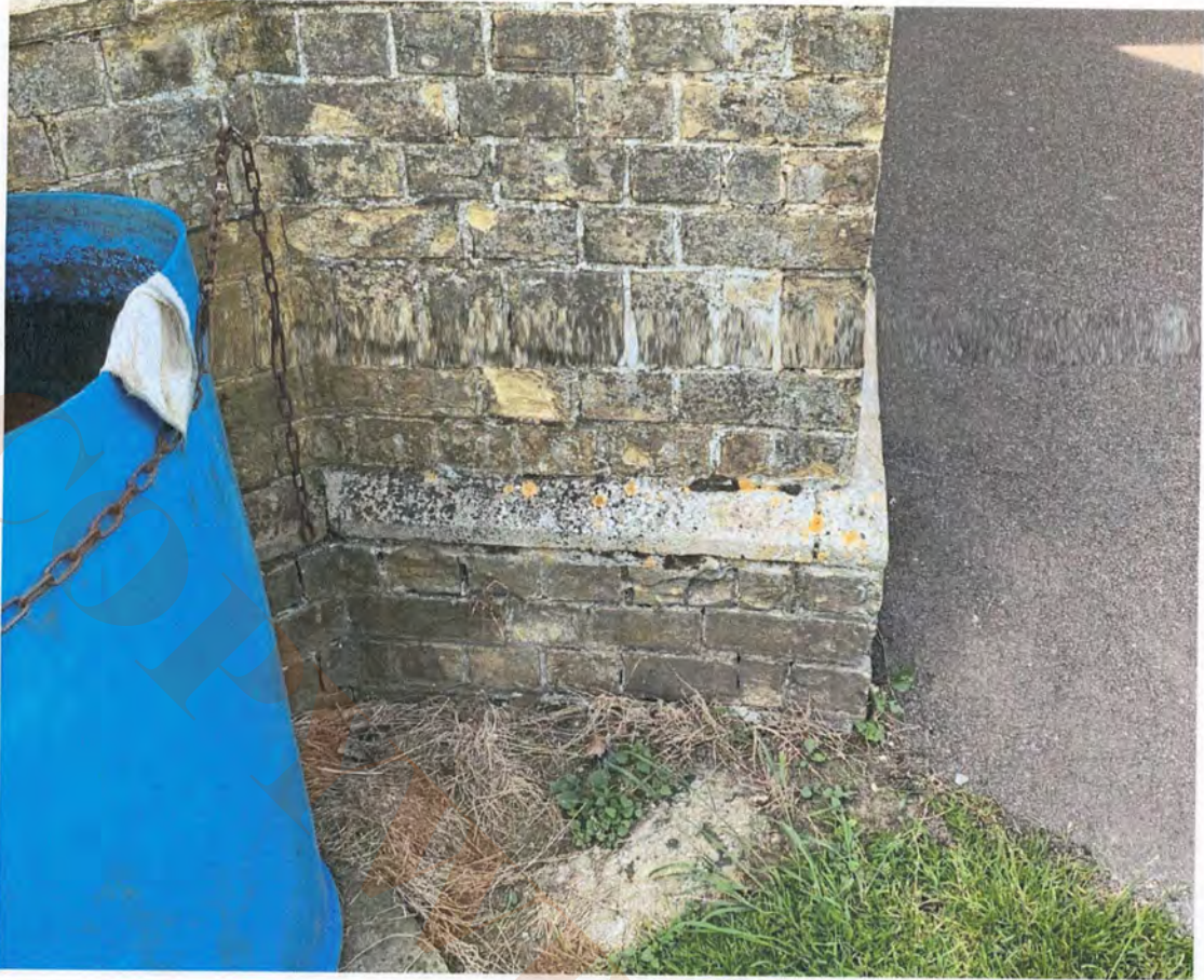
8.42 South chapel north east buttress
