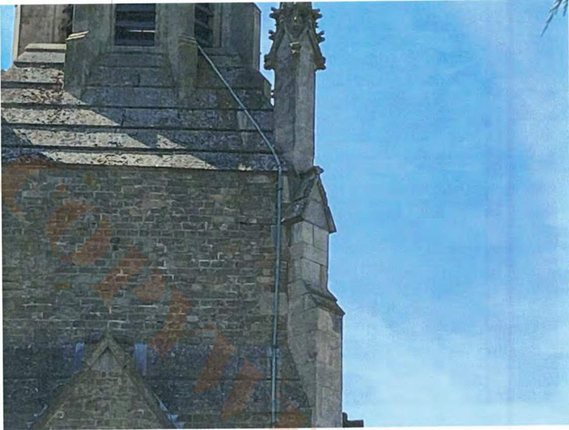
8.1 Tower north east buttress 8.1 Tower walling
