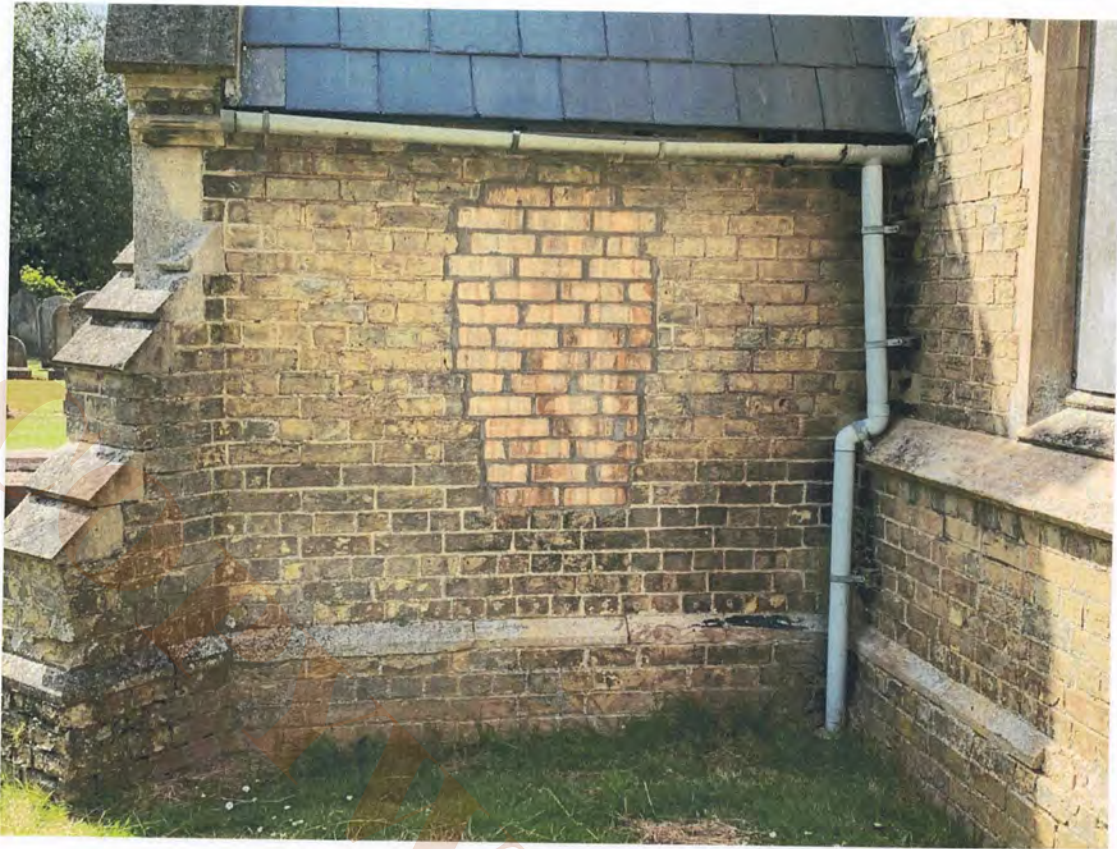
10.12 South porch rainwater goods east eaves
