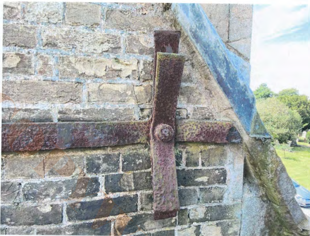
8.2, 8.3 Tower north elevation ironwork
