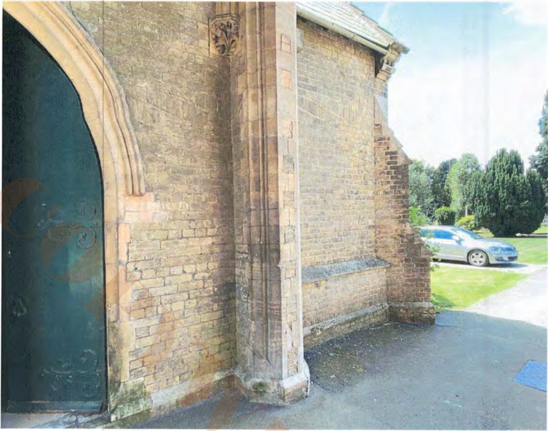
9.10, 9.11, 9.12 Tower west elevation south pier
