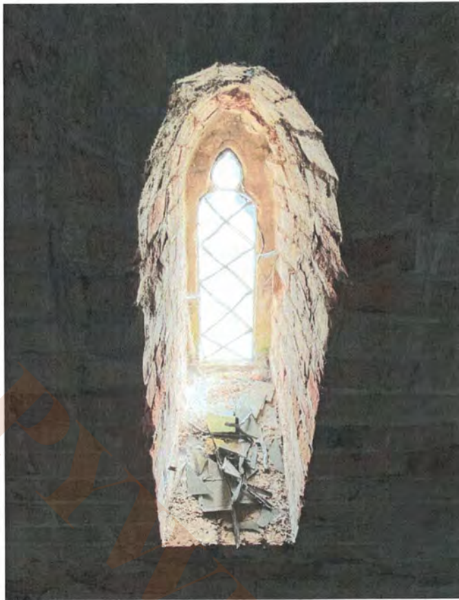
9.3 Tower east window (internal view)
