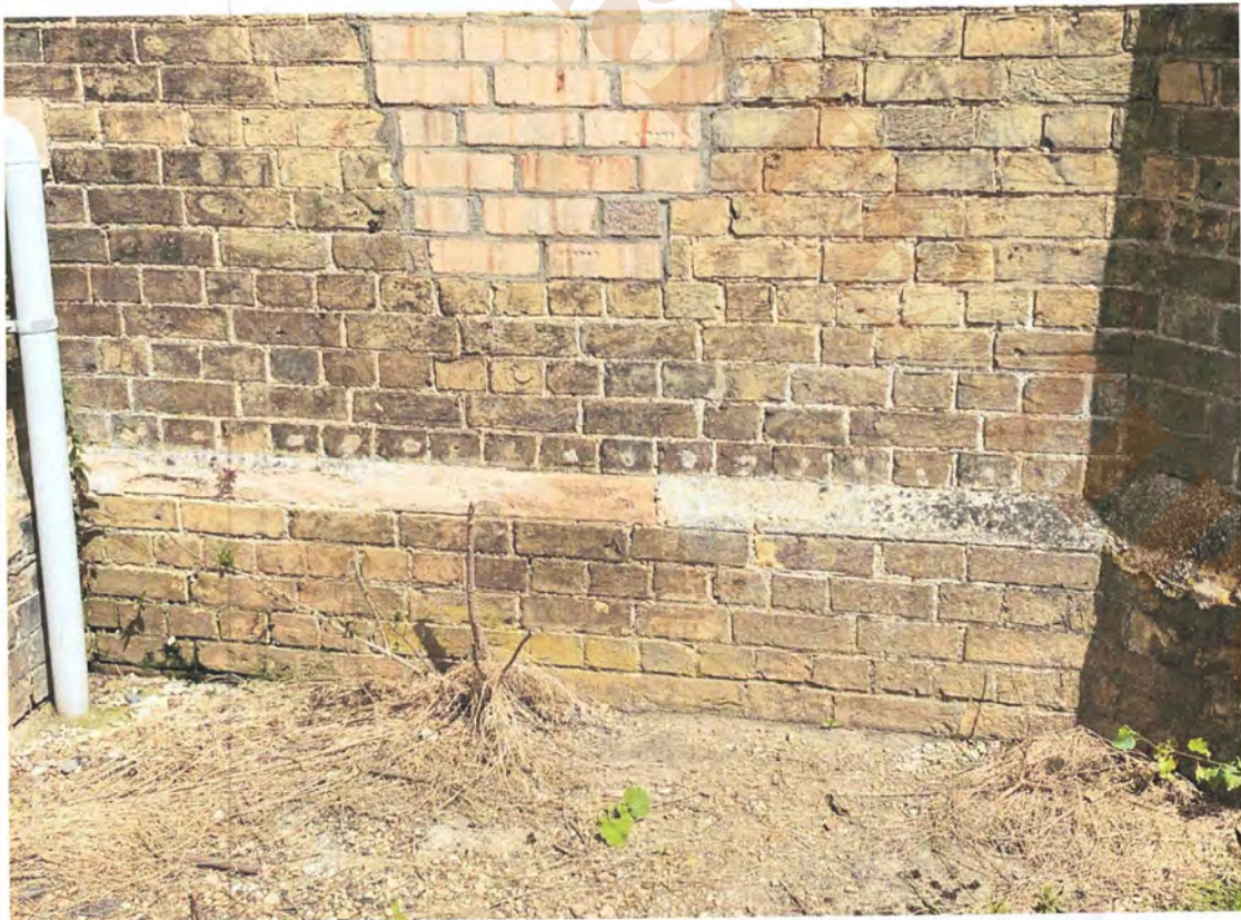
8.61 South porch west elevation
