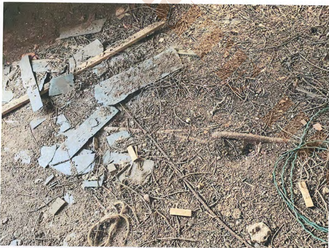
11.4 Tower lower chamber floor
