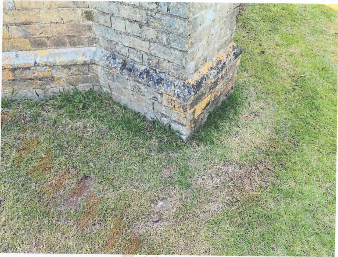
8.20 North elevation north east buttress
