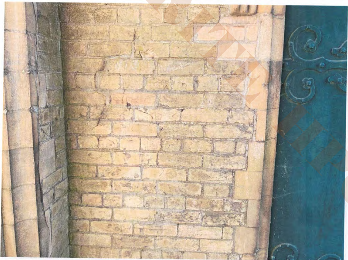
11.13 Carriageway south wall east
