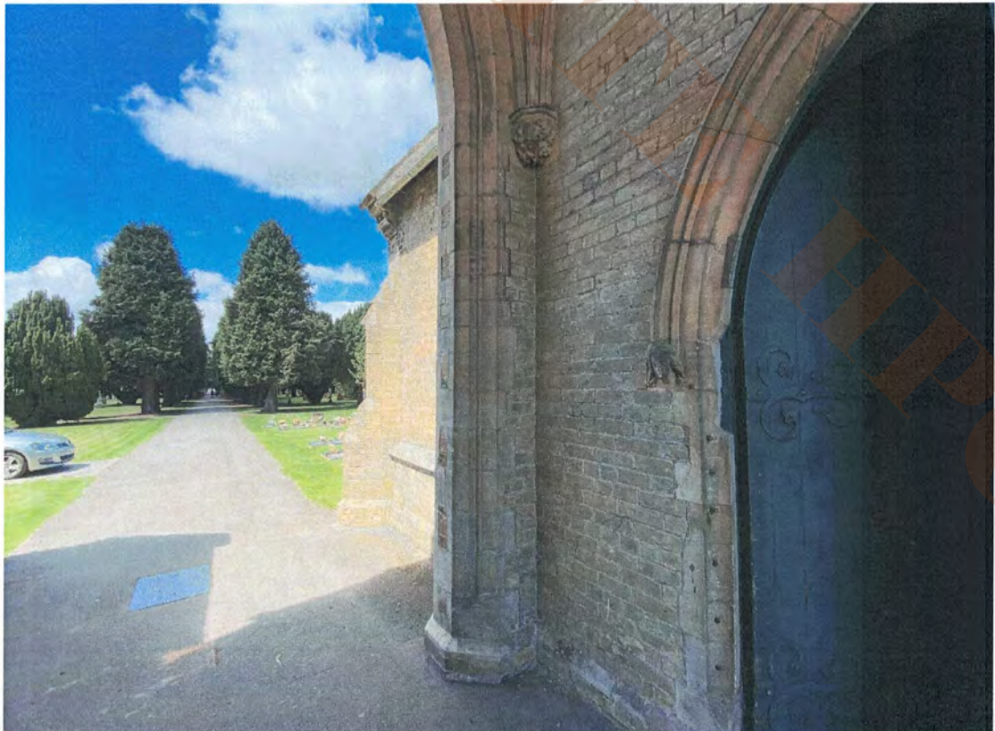
9.9 Tower west elevation north pier
