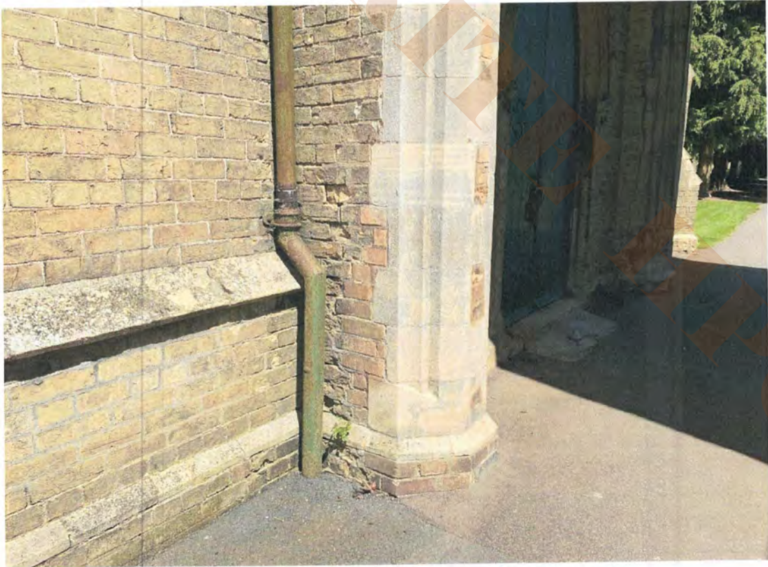
8.16 West elevation north pier
