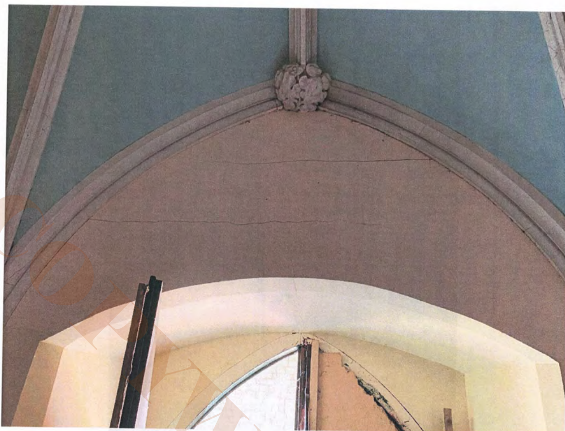
11.21 South chapel north wall
