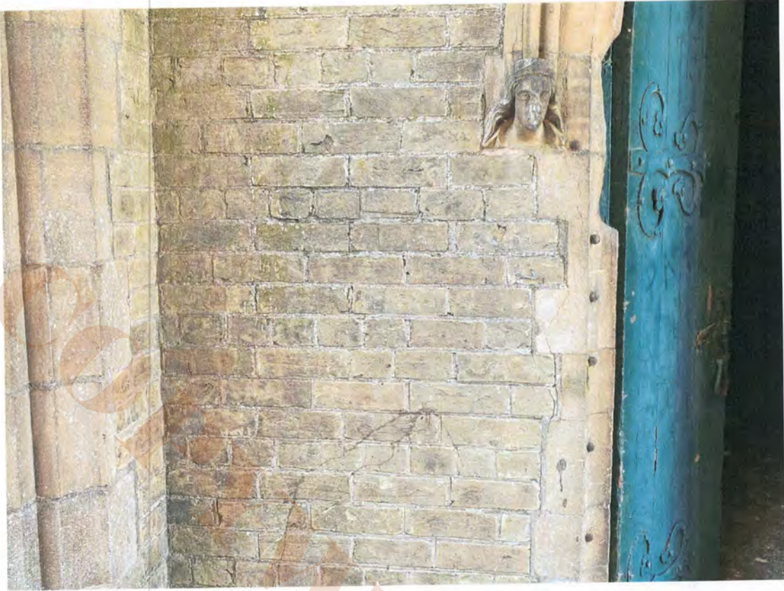
11.9 Carriageway north wall west
