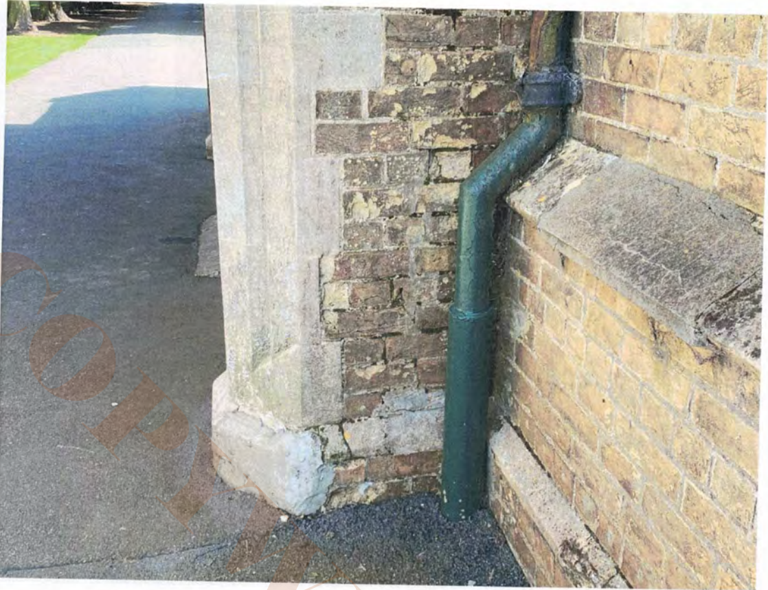
8.16 West elevation south pier
