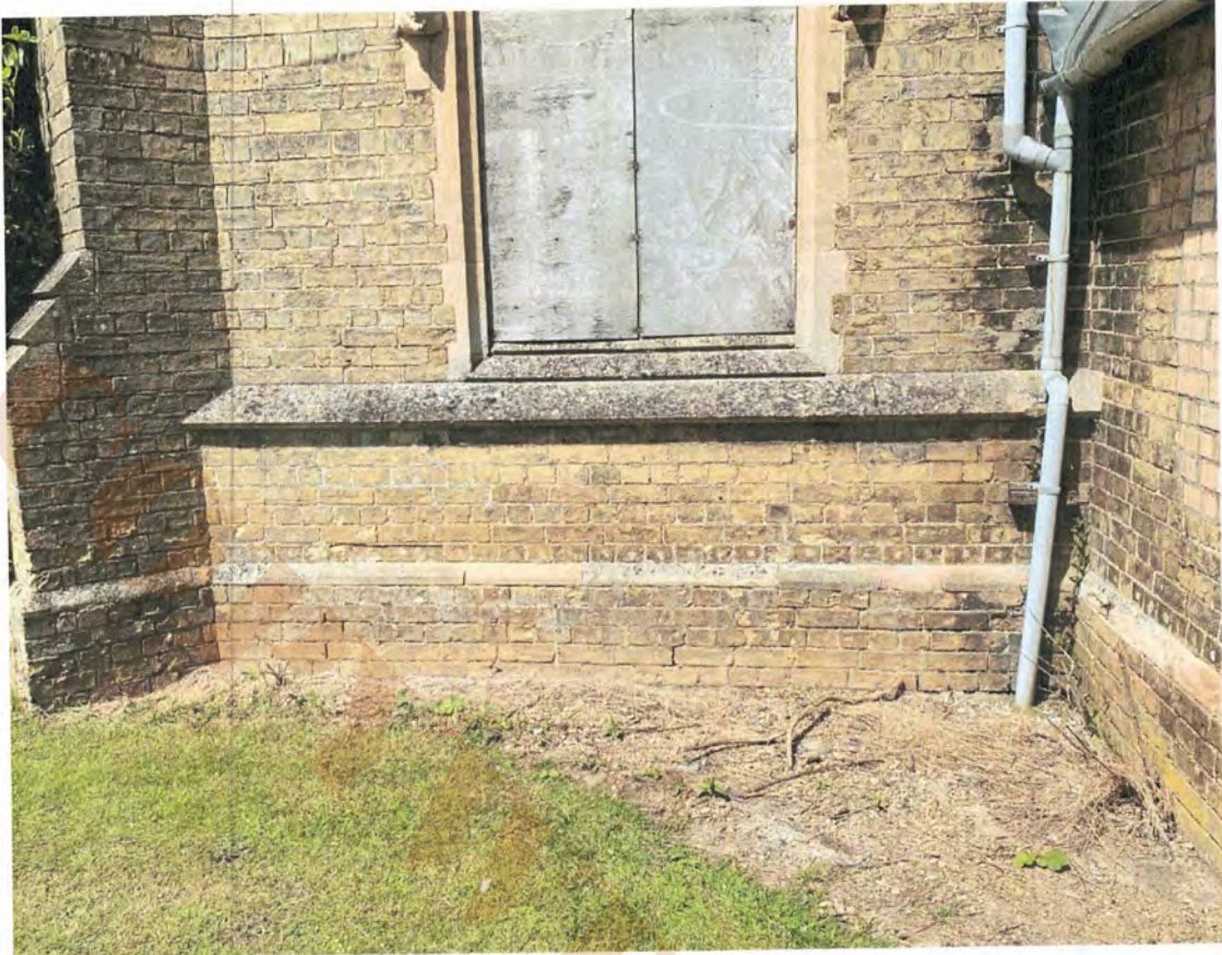
8.49, 8.50 South chapel south elevation west of porch
