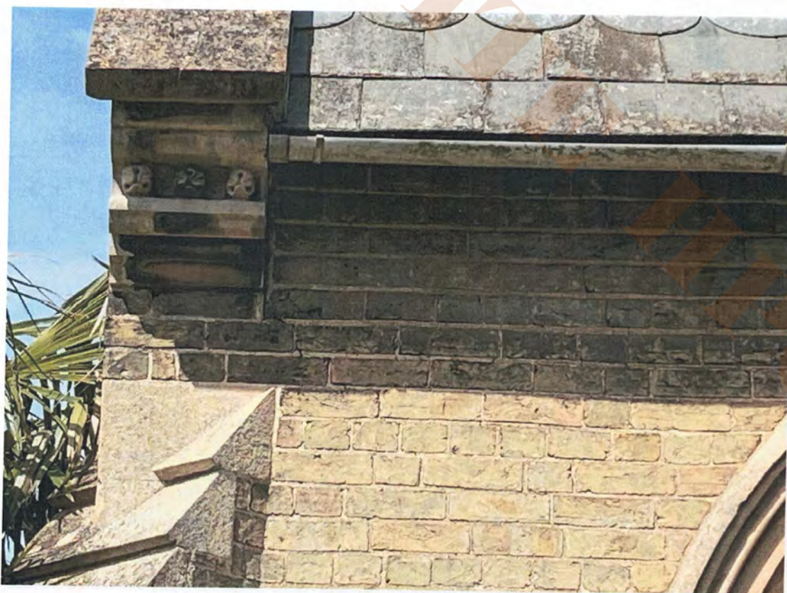
8.48 South chapel south elevation west of porch
