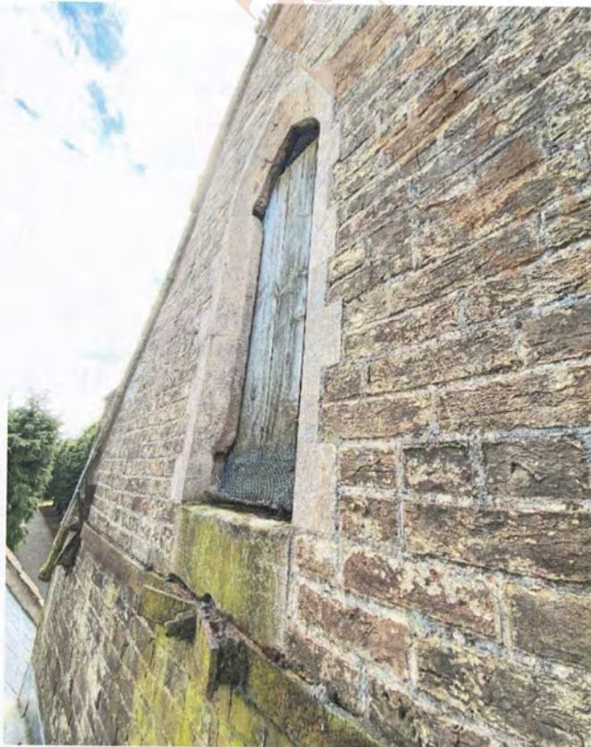
9.2 Tower north door
