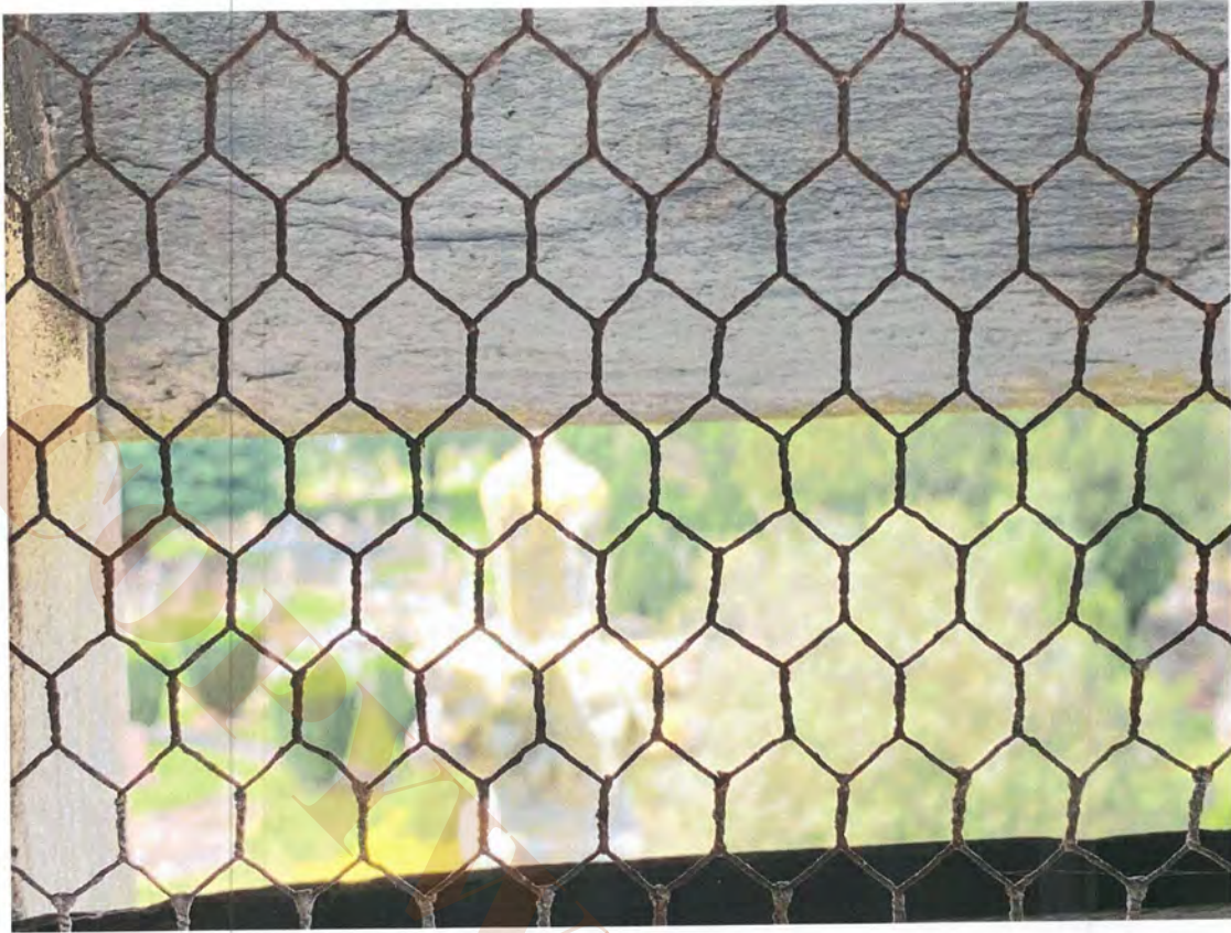
11.2 Tower interior mesh
