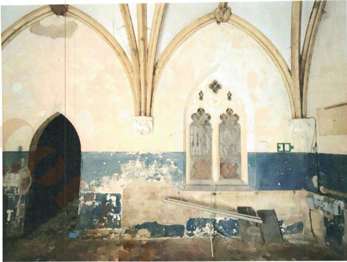
11.36 North chapel north interior
