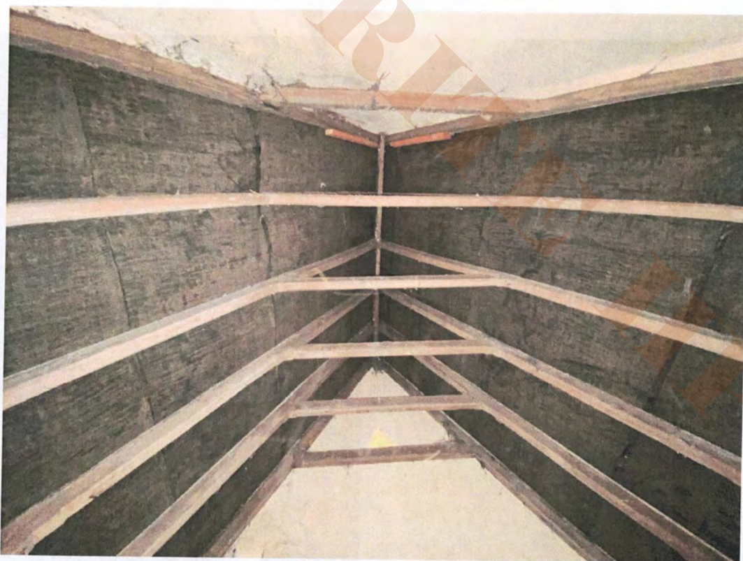
11.29 North porch ceiling
