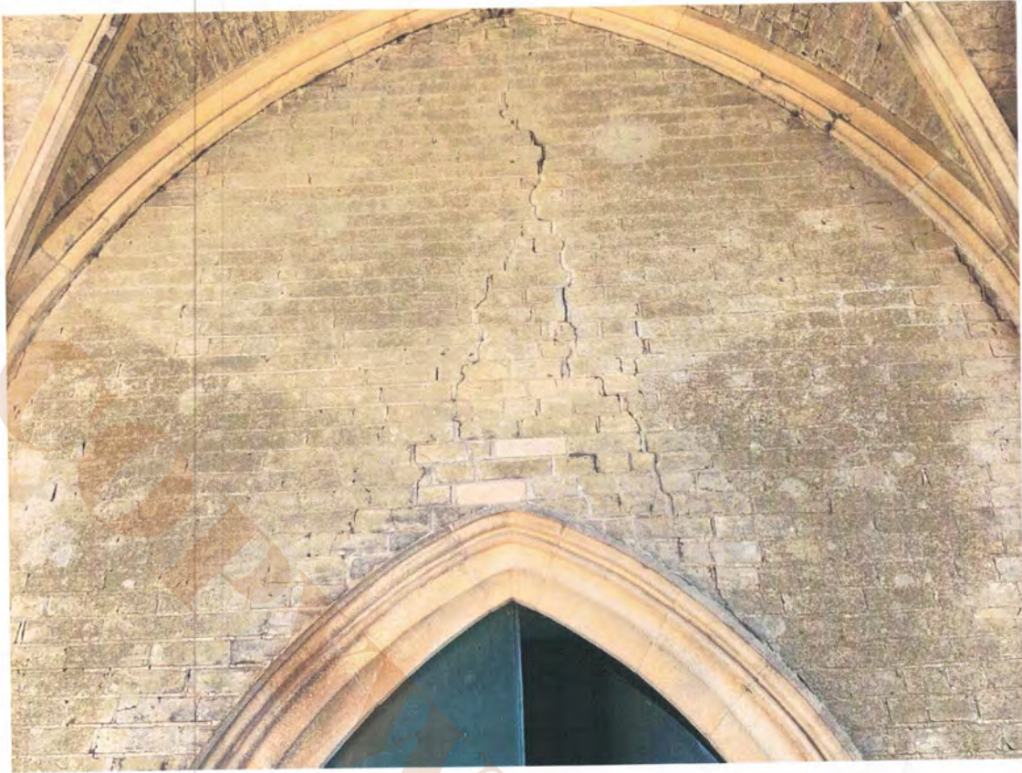
11.14 Carriageway south wall
