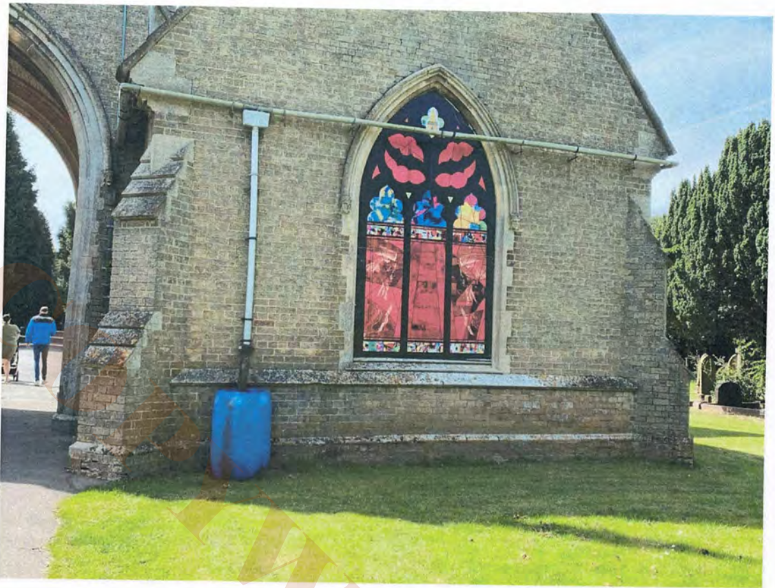
10.3 North chapel rainwater goods on east elevation
