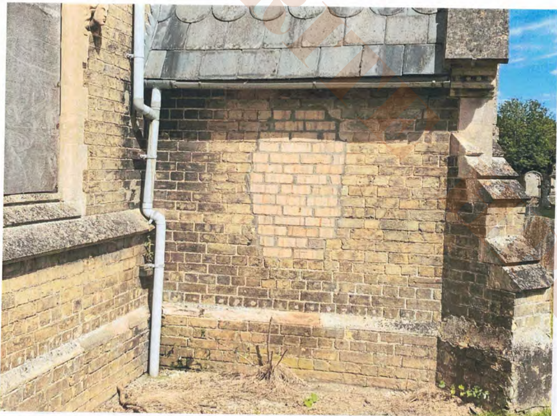
10.13 South porch rainwater goods west eaves
