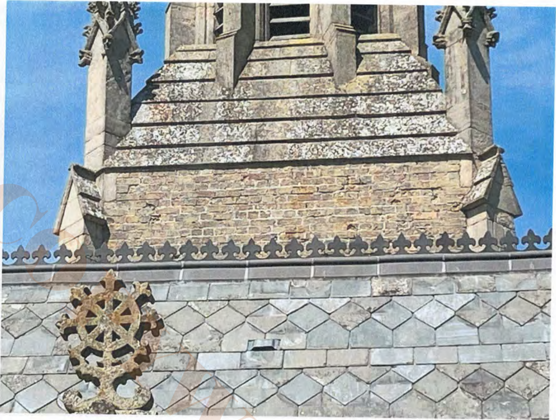
8.10 Tower south elevation seen over chapel roof
