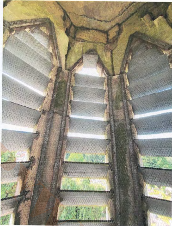
9.1 Spire louvres (typical, internal view)
