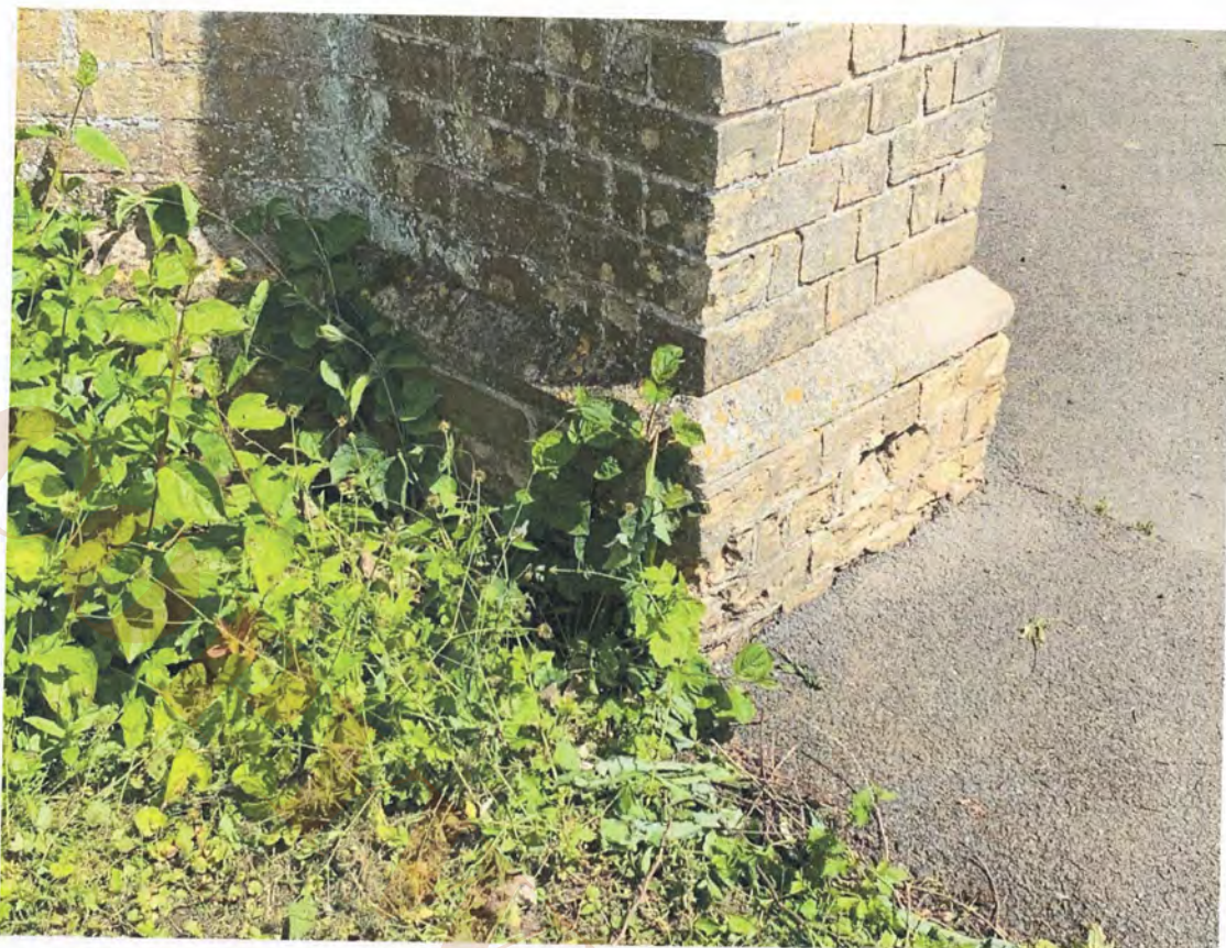
8.27 North chapel south west buttress
