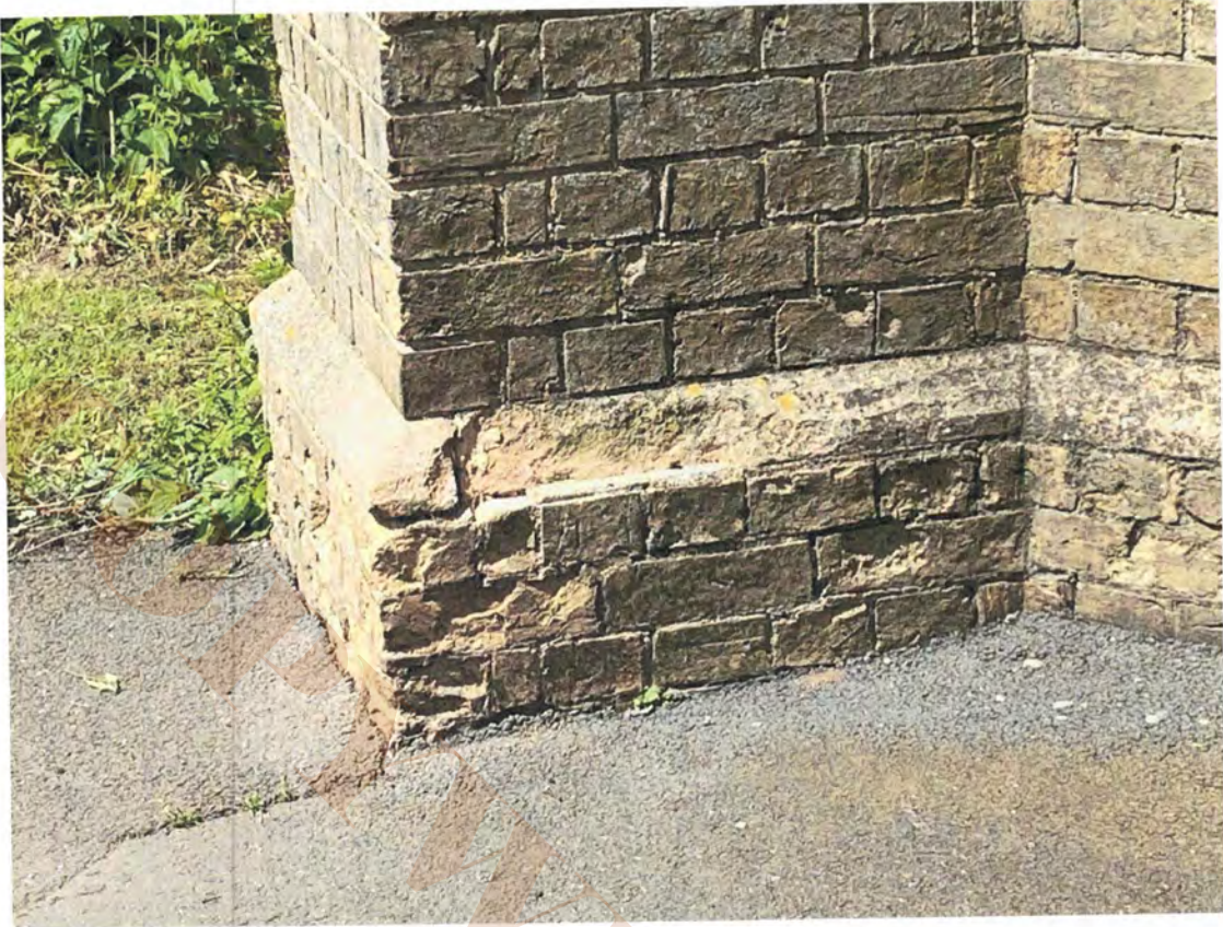
8.24 North chapel south west buttress
