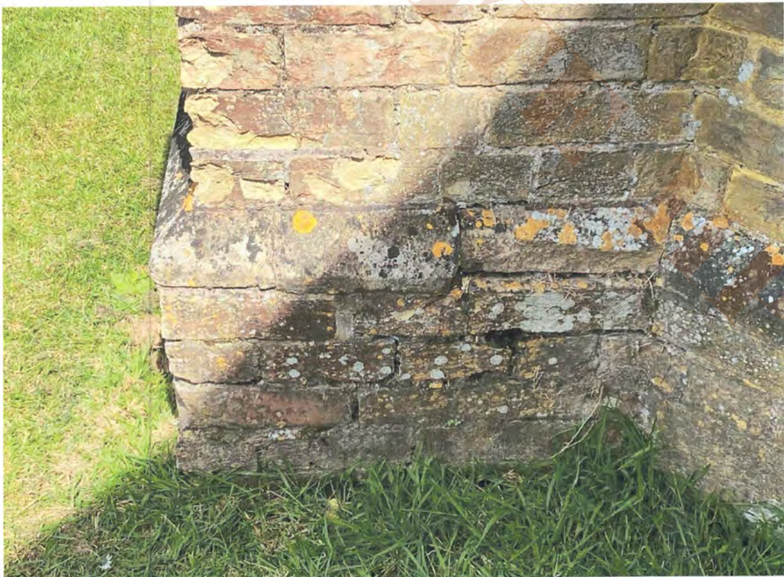
8.34 North porch north west buttress
