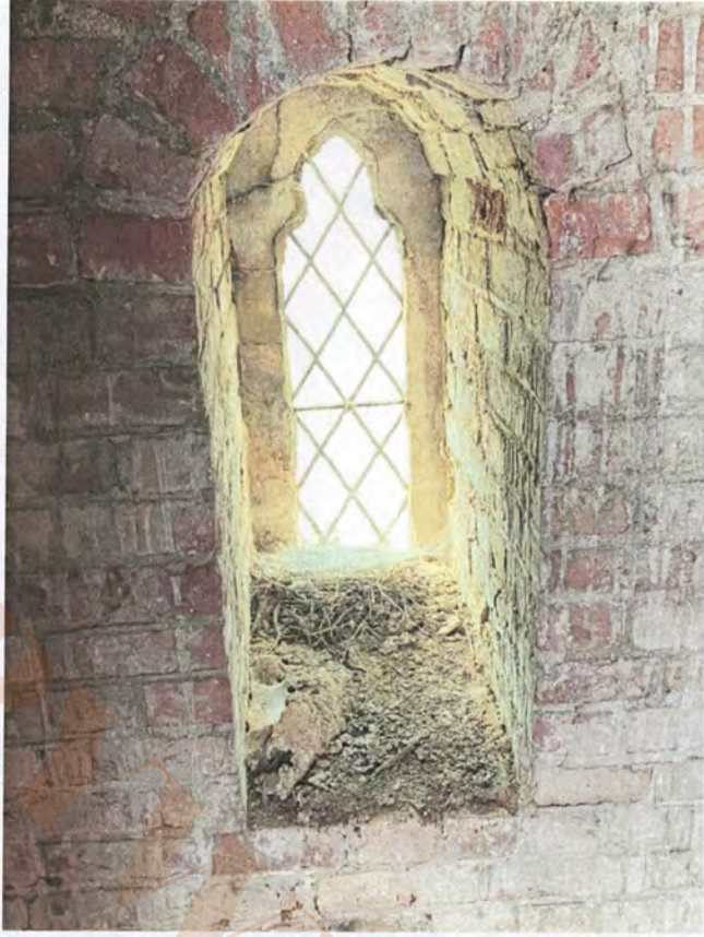
9.4 Tower south window (internal view)
