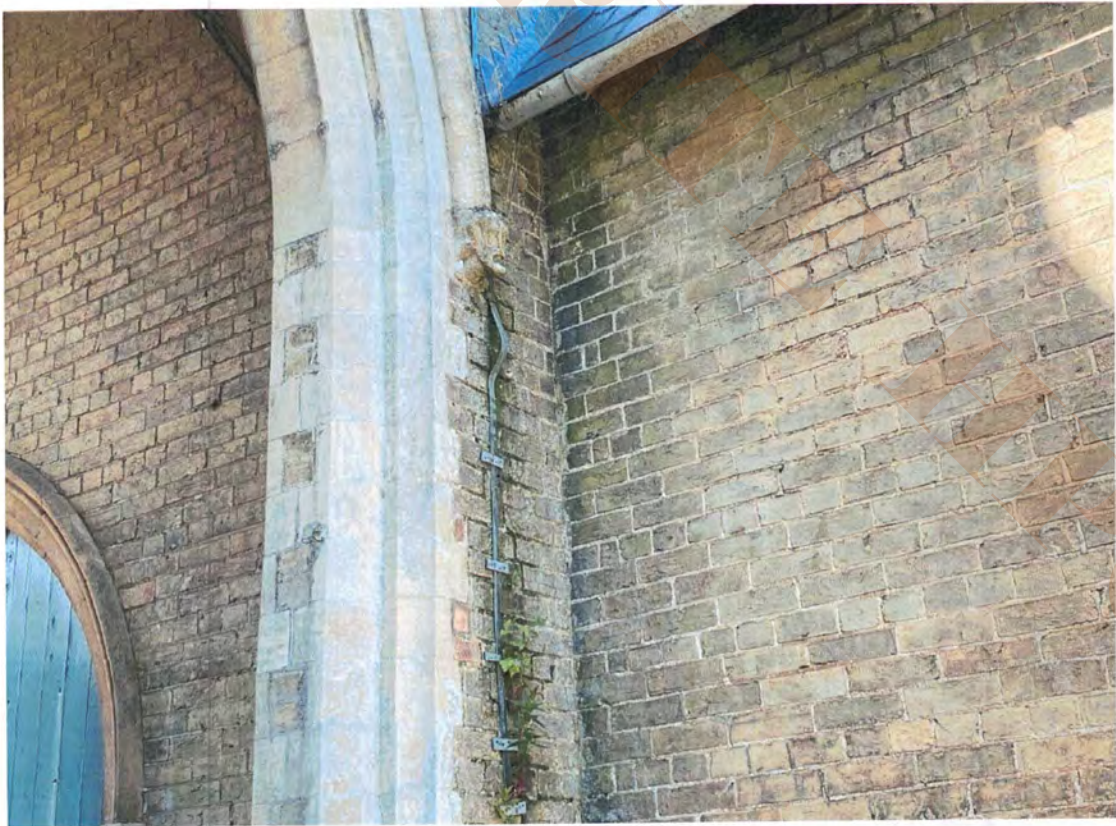
8.8 Tower east elevation north side brickwork
