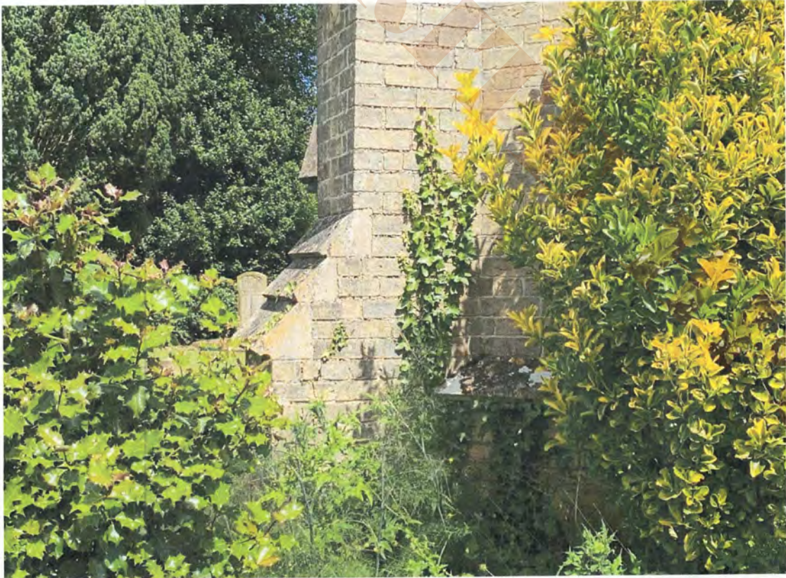
8.29 North chapel west elevation ivy
